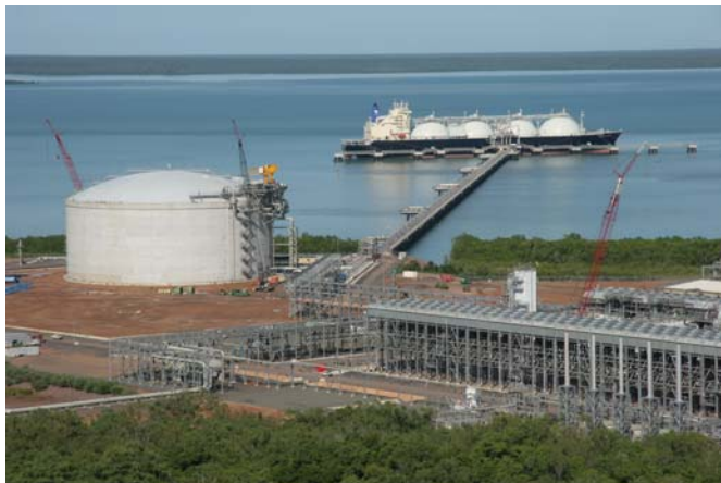
A Japanese gas carrier loads at the Darwin LNG Plant at Wickham Point.
